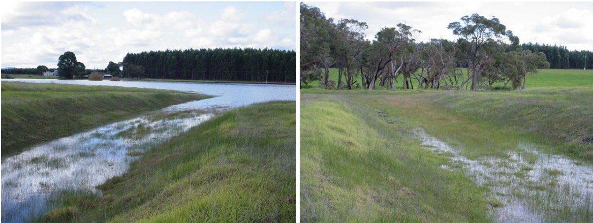
Figure 5 Main storage dam spillway during overflow July to October 2005.
