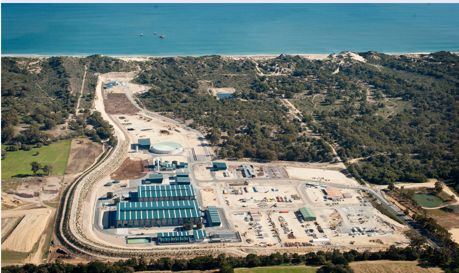
The Southern Seawater Desalination Plant has won a number of awards this year, including the overall WA Engineering Excellence Award.
