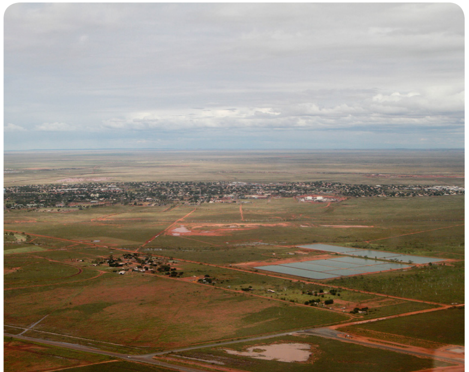
There are a number of infrastructure projects in the North West which will be available for tender in the next year.
