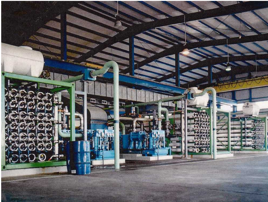
Figure 3: Rack with RO modules
