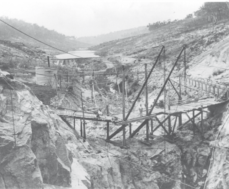
MUNDARING WEIR CONSTRUCTION, 1898-1903 FOUNDATION OF WEIR WALL LOOKING EAST
