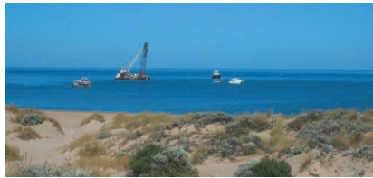
View over the marine construction zone
