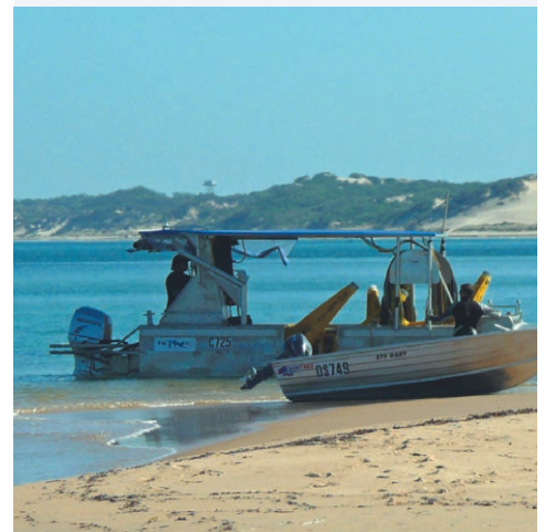
Contractors preparing to install the marine marker buoys
