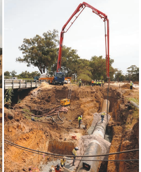
SSDP Trunk Main river crossing
