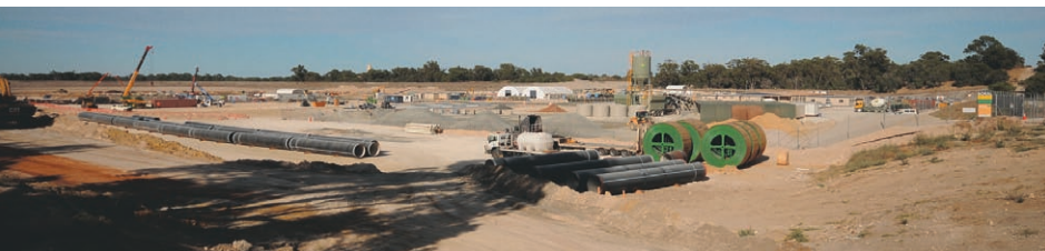
Plant site taking shape
