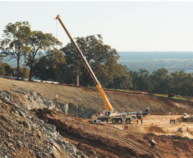
View looking west over the tank site.
