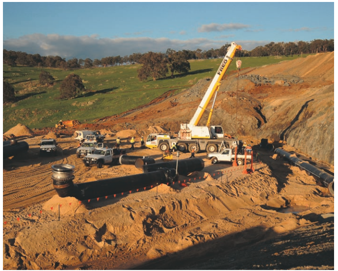
Pipe laying commences at the site.
