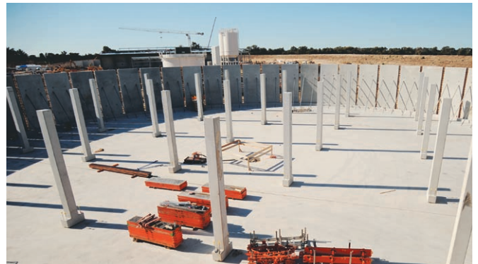
Drinking water tank.
