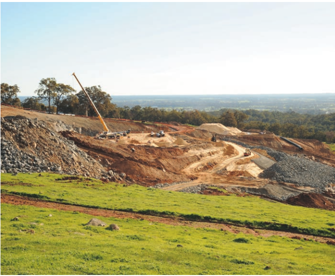
View over the tank site.
