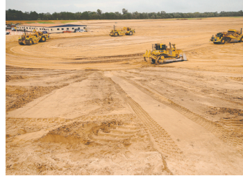
Plant site earthworks underway.
