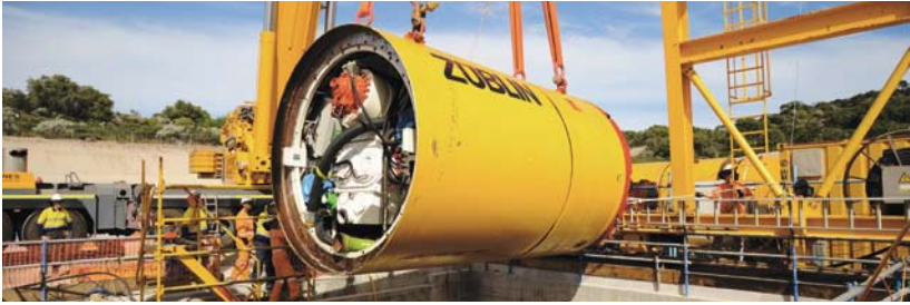
Tunnel Boring Machine used to tunnel under the dunes and beach.
