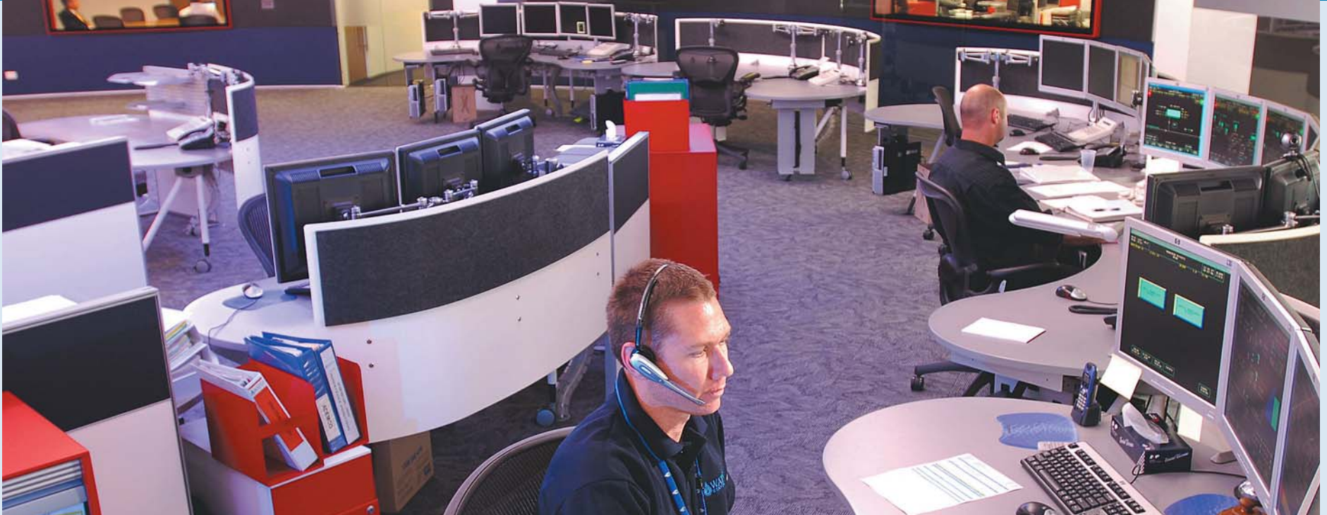
When there are faults or emergencies, alarm signals from monitoring equipment installed on Water Corporation assets are relayed to a central monitoring point, which is staffed 24-hours-a-day, seven-days-a-week.
