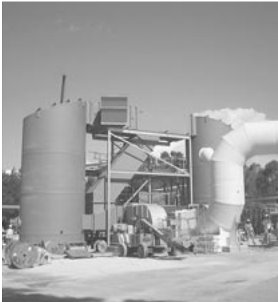
New scrubbers in place.
