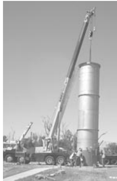
Installing the new gas flare.
