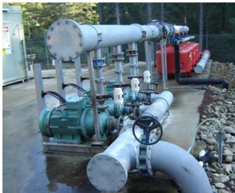
Recycled Water Pump Station at Margaret River Wastewater Treatment Plant
