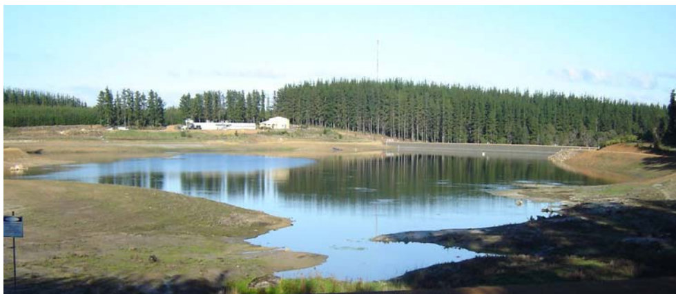
Margaret River Wastewater Treatment Plant and Storage Dam
