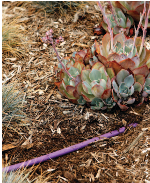
Greywater system and lilac dripline in a home garden
