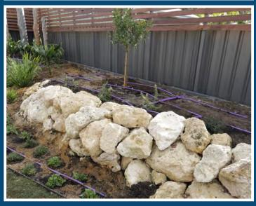
also been included at the highest point of the irrigation line. This allows air to enter through the one-way valve as the water drains out of the line avoiding the potential for dirty water being sucked back through the drippers that can lead to them becoming blocked with grit. Greywater irrigation drip lines are setback from paving, retaining walls, neighbouring properties and buildings to comply with the Code.
