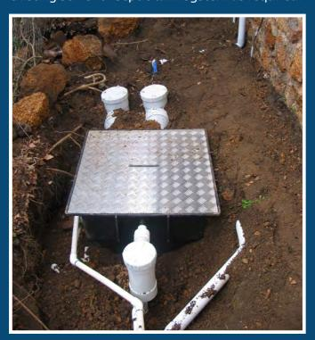
Cleaning of the filter should occur fortnightly or weekly if excessive laundry and bathroom use has occurred. This device redirects wastewater from the existing system to a disconnector gully return or directly to sewer via a reflux valve.
