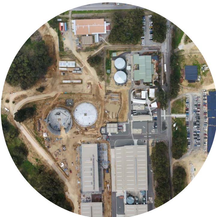
Construction of Stage 2 Groundwater Replenishment Scheme
