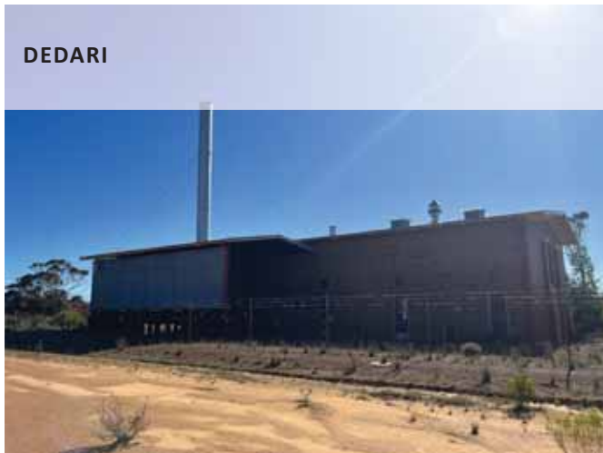
NO. 8 PUMP STATION
