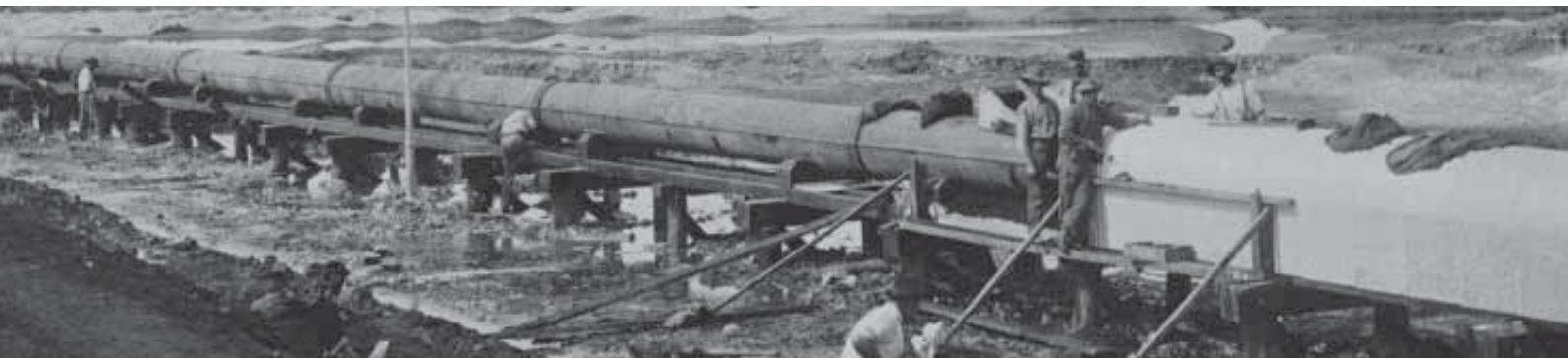
Image 23: Construction process of the GWSS
