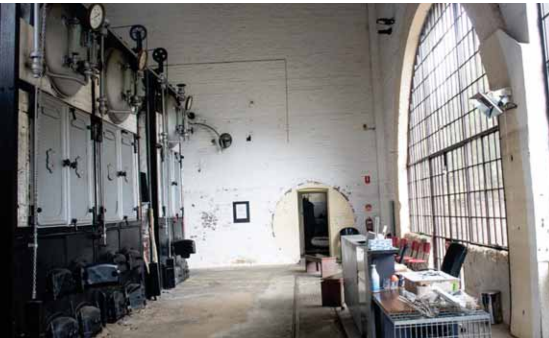
Image 15 +16: Interior of Pump Station 1 Museum with Babcock and Wilcox water tube boilers
