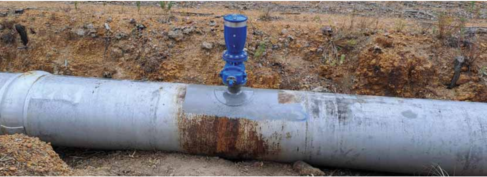
Image 59: GWSS, new air valve at Bakers Hill
