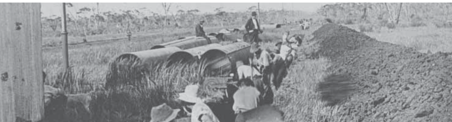
Image 26: Digging a trench to lay pipes for the GWSS
