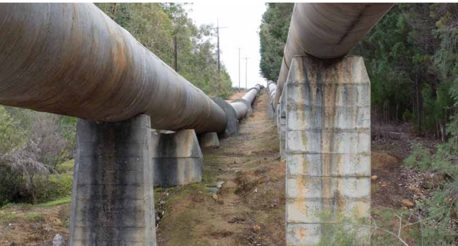
Image 52: Anchor blocks and stabilisation at Fred Jacoby Park
