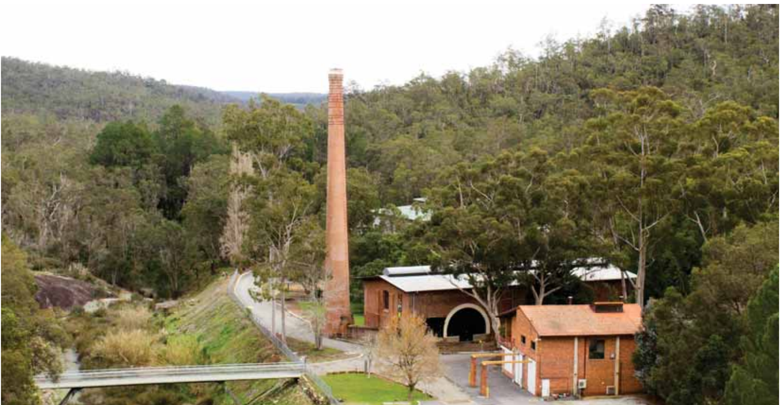
Image 12: Place No. 1 Pumping Station
