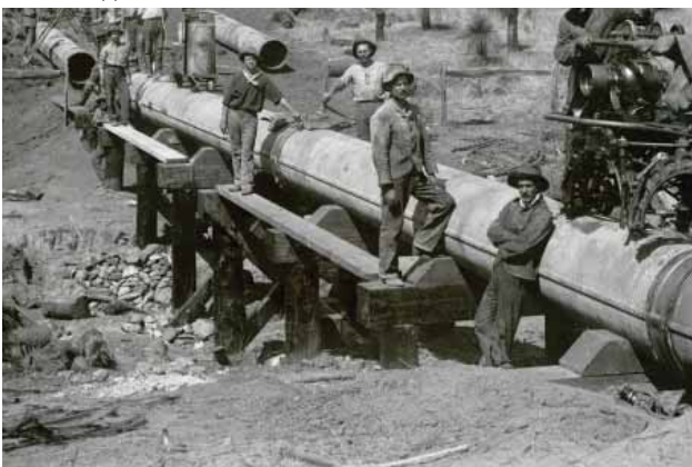
Image 25: GWSS pipe and caulking machine
