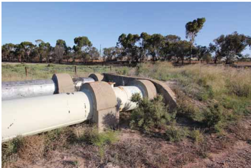
Photograph 01 Locking bar pipeline emerges from ground near Meckering Griffiths Architects, April 2016
