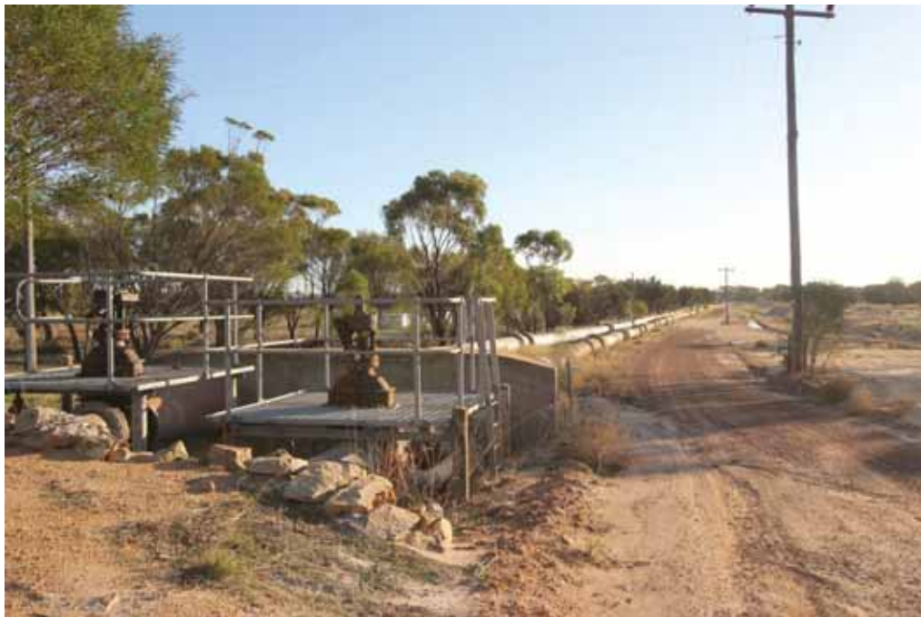
Photograph 04 GWSS goes below ground by the Meckering booster pump station Griffiths Architects, April 2016
