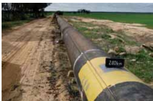
Section of locking bar pipe near Burracoppin (2014)
