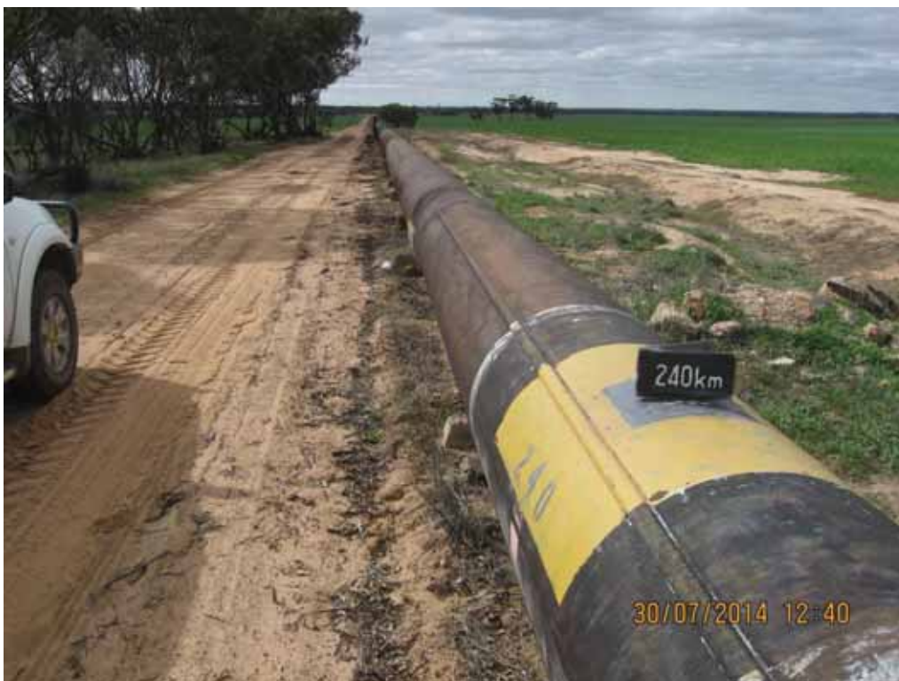
Photograph 06 Locking bar pipe near Burracoppin Water Corporation, July 2014
