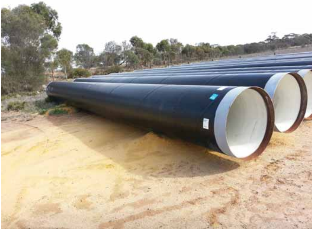
Photograph 13 Spiral weld MSCL with plastic coating before being laid below ground Water Corporation
