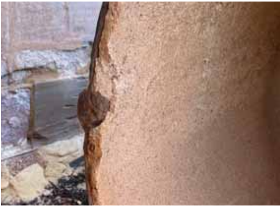
Image 8: Close up of cross-section of locking bar pipe
