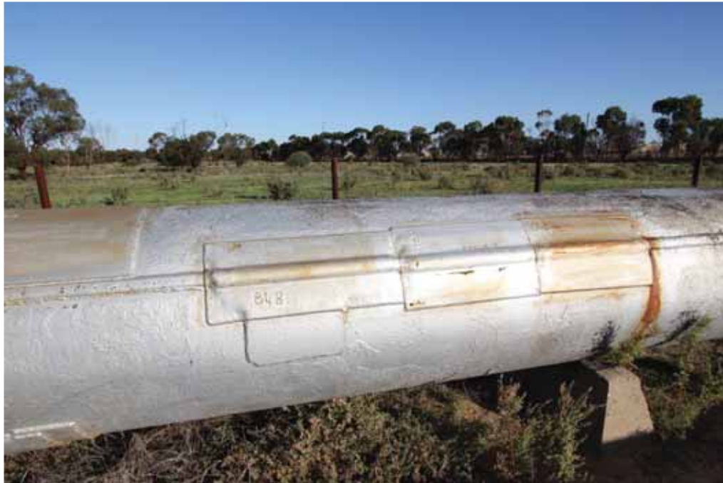
Photograph 03 Repairs to locking bar pipe near Meckering Griffiths Architects, April 2016
