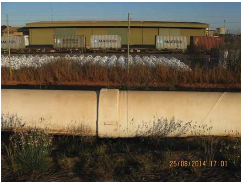
Photograph 14 Locking bar meeting spiral weld MSCL pipe Water Corporation, August 2014
