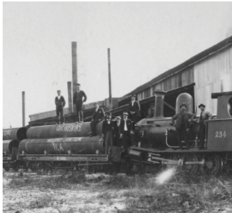
Image 36: Initial Pipes for the Pipeline Leaving Midland
