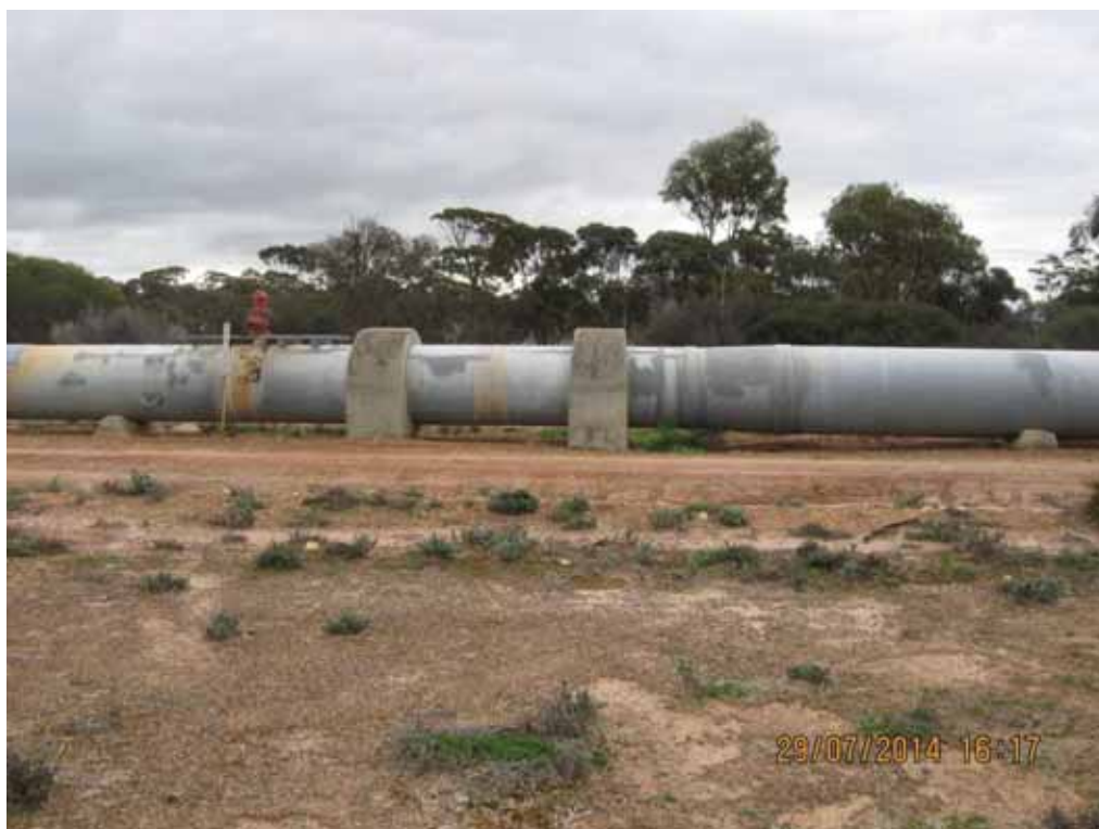
Photograph 08 MSCL pipe Water Corporation, July 2014
