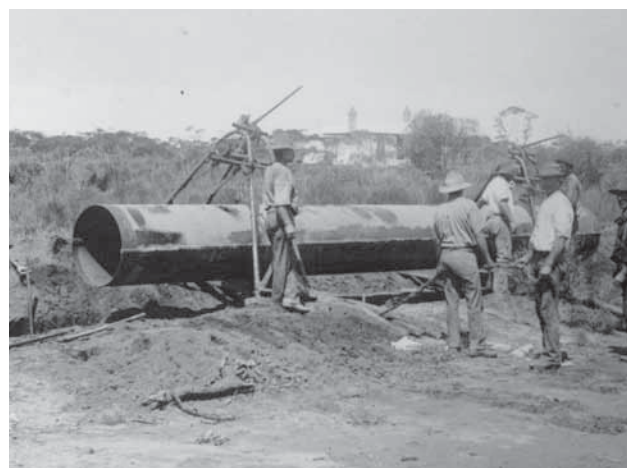
Image 22: Pipe Lowering near Kalgoorlie
