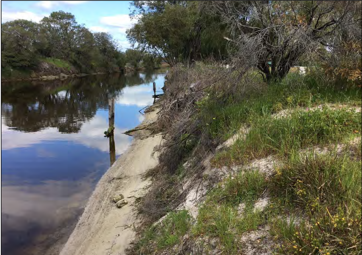
VDD Embankment - September 2020
