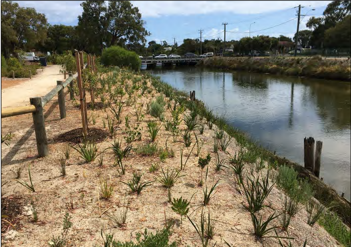
VDD Embankment - December 2021
