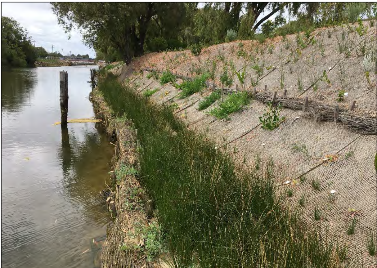
VDD Embankment - December 2021
