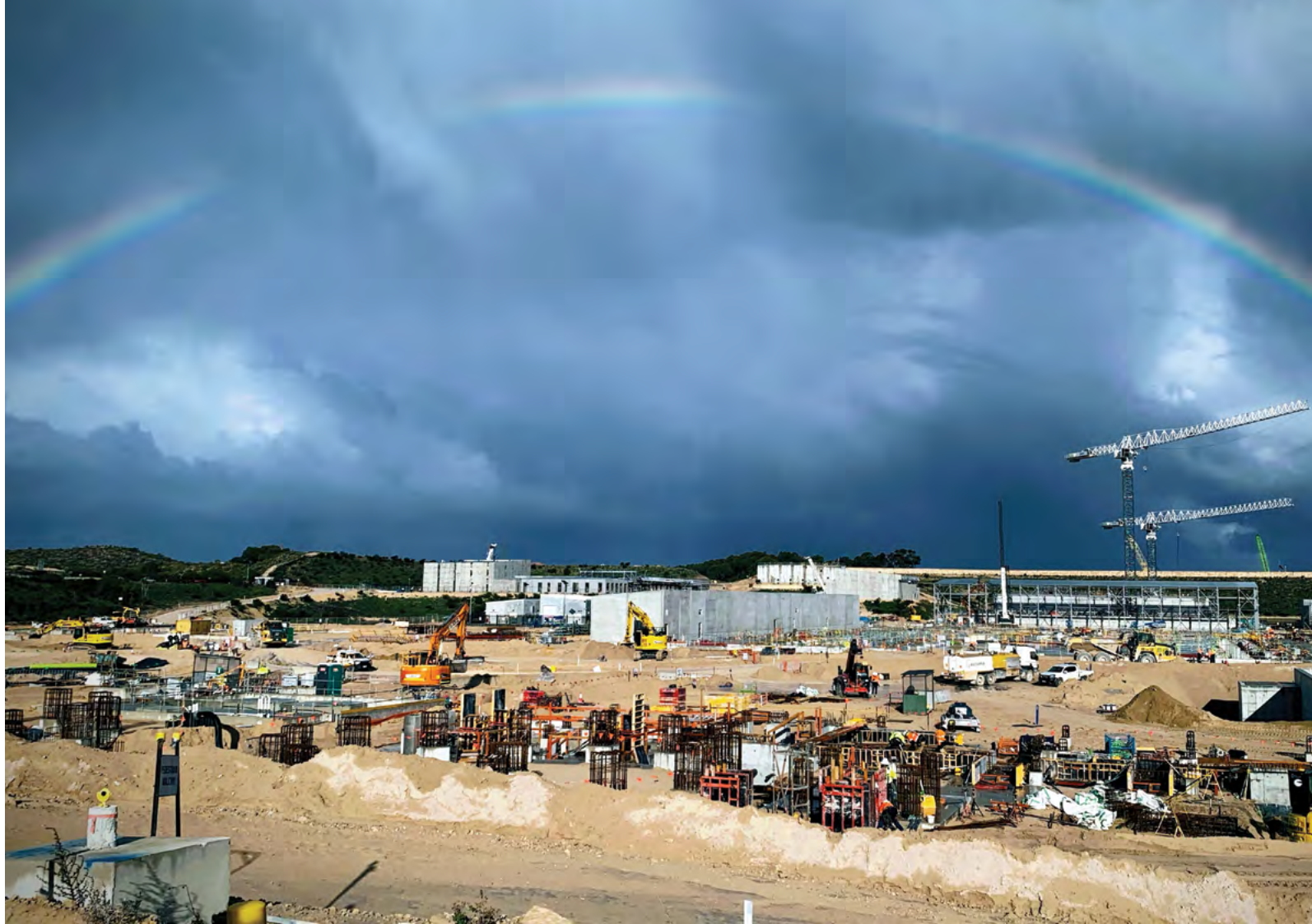
A rainbow appears over the ASDP construction site.
